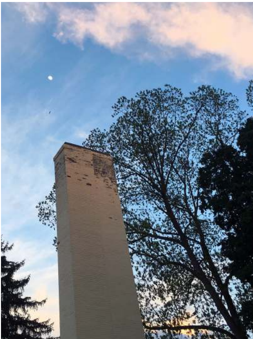
The Knutti Boiler Chimney
